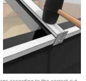
screws. Repeat for all the rafters. Note: Drill an additional 5mm hole and add a pressure plate screw. Always add a pressure plate screw through the pressure plate in line with the double-sided tape to help compress the glass to the tape.
