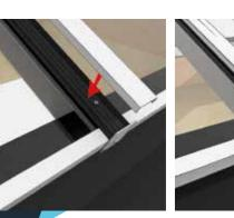
Fit all the rafter topcaps according to the correct cut length and roof plan position. Locate over the top of the pressure plate and push down. A rubber mallet may be required.
