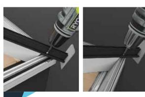
Fix hips into ringbeam using the provided 4.2 x 25mm fixings on either side of the rafter as shown.
