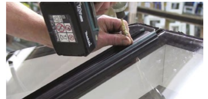
6 Position the plastic central pressure plate over rear rafters and fix with screws.
