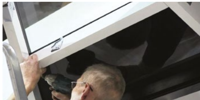
4 Screw fix the upper ringbeams through the pilot holes provided into the side of the hip rafter.
