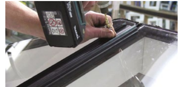
2 Fit remaining pressure plates into position.
