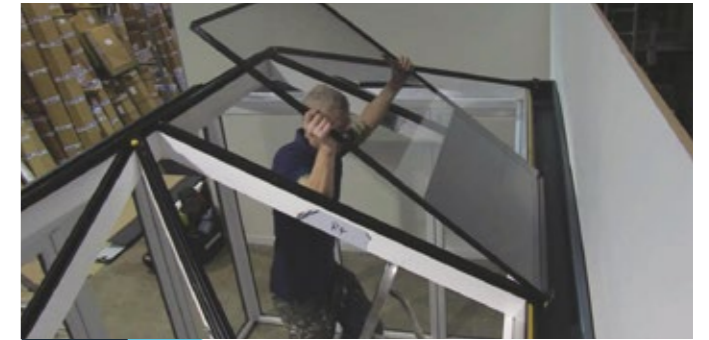
4 Lift glass into place behind the rafter end stops and press down glazing. Make sure the protective yellow tape is removed.
