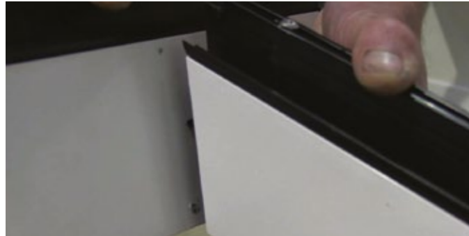
7 Place the rafter into the slot on the ridge and slide the rafter up.
