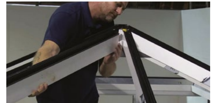
4 Slide the hip rafter over the bracket and push it tight against the ridge.
