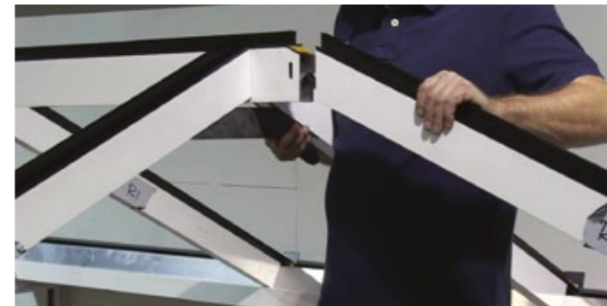
3 Fix the opposite ridge end rafter.
