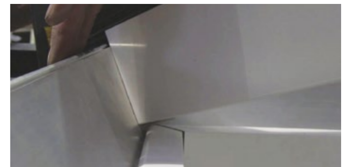
6 Rotate the ringbeam flaps keeping them tight against the hip rafter cut before fixing.
