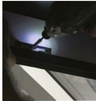
3 Fix the hinge attached to the ladder frame onto the inside of the upper ringbeams. Make sure ladder frames are level before securing.
