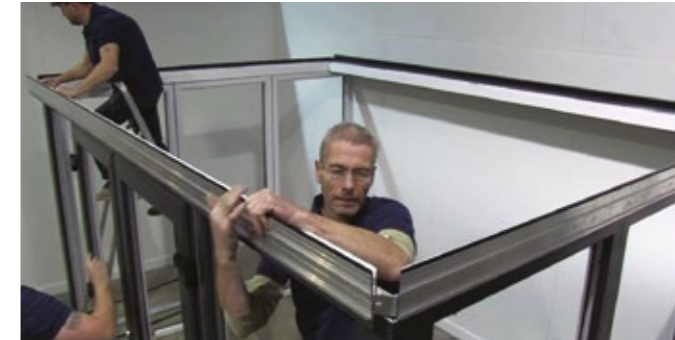
7 Lift the final front ringbeam into position and slide the ringbeam bracket into the channel on the
