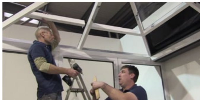
5 Fit the remainder of the upper ringbeams into position.
