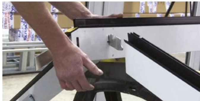
9 Fix remaining rafters on the main A-frame.
