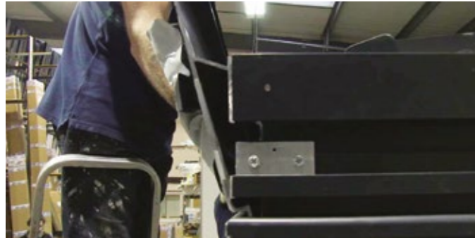
1 Lift the external cornice into position by positioning them at the bottom edge of the aluminium gutter and let them drop into place (see Figure 4).
