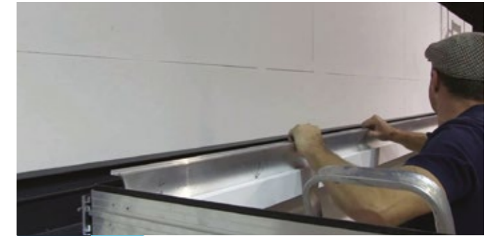
10 Position the ringbeam flaps into place. Flap engages at approximately 90°.
