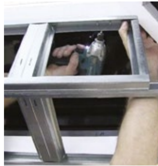
3 Fix the hinge attached to the ladder frame onto the inside of the upper ringbeams. Make sure ladder frames are level before securing.
