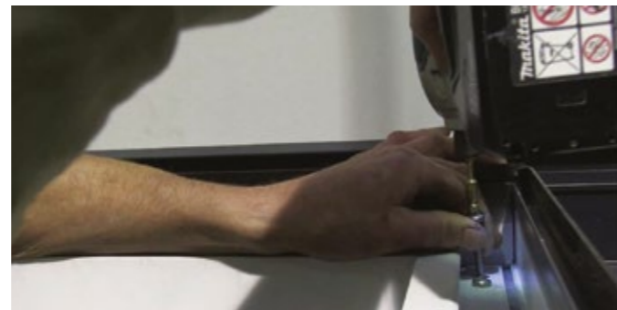
6 Fix the ringbeam screws into predrilled holes from above.
