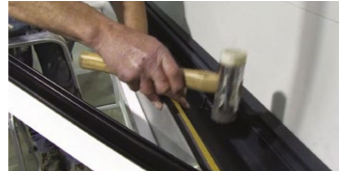
1 Once rafters are fixed, remove the foam boards and locate the glazing shelf.
