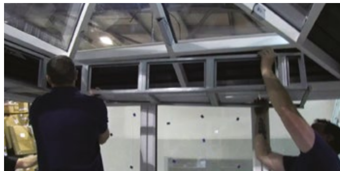
5 Fix the remainder of the ladder frame making sure the internal corners are securely fitted.
