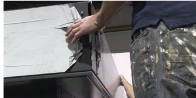
2 Fit remainder of cornices.
