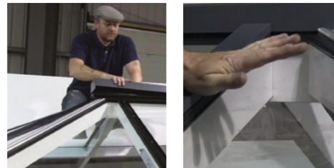
5 Position the ridge cover cap over the ridge pressure plate and clip down securely. Clip on the external cover caps.
