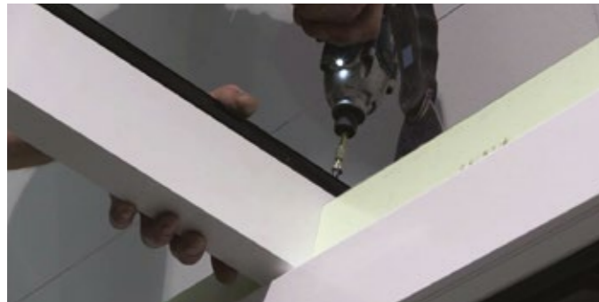
9 Once the rafters are in position pull the ringbeam flap up tight to the rafter and fix centrally with a screw (see Figure 2).
