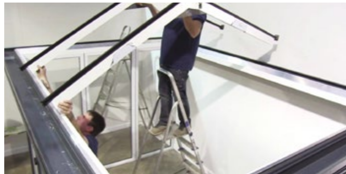
10 Lift the main A-frame into position.
