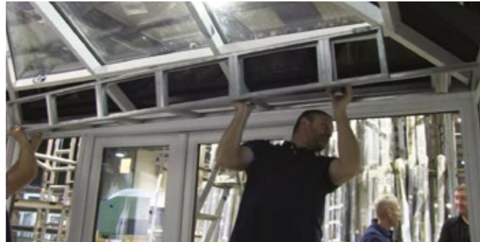
2 Lift the longer ladder frame into position between the ringbeams.
