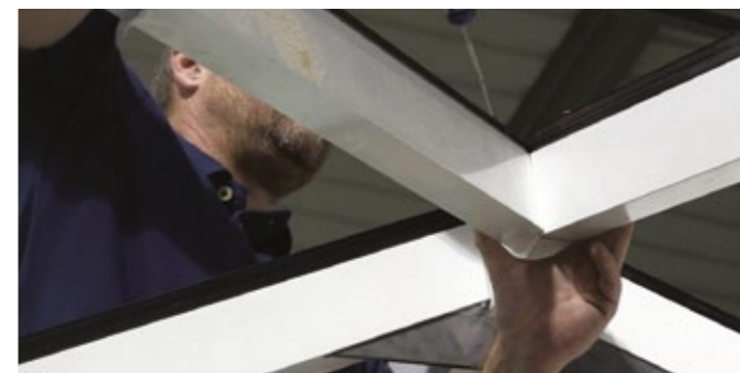
5 Secure the hip rafter by fixing the top screw.
