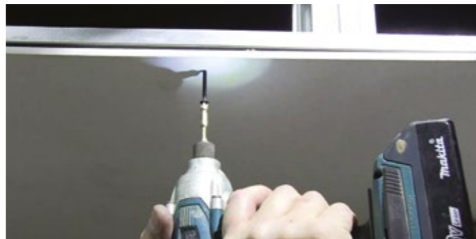
6 Screw plasterboard into the steel ladder grids.
