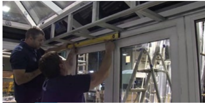
4 When frames are level fix the ladder frame to the back of the ringbeam (see Figure 5).
