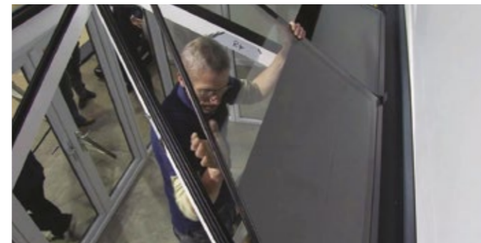
5 Fit all the rear units of glass keeping the glazing end closer between the rafters.
