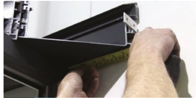
4 Centre the gutter on the frames.
